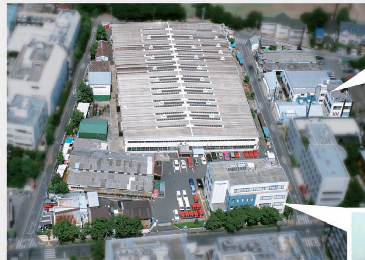
Old Tokyo Plant
